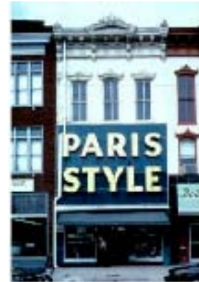
Example of bad wall sign – not permitted
