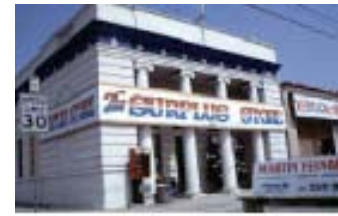
Example of bad wall sign – not permitted
